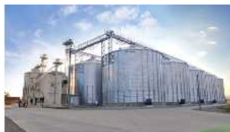
Grain drying facility
